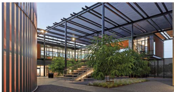
Central Energy Facility Chiller Plant Expansion
